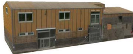
Texture components and the 3D-Model derived from UAV images of the HXE-building at Campus Science City Campus ETH Hoenggerberg, displayed in VRMLVIEW
