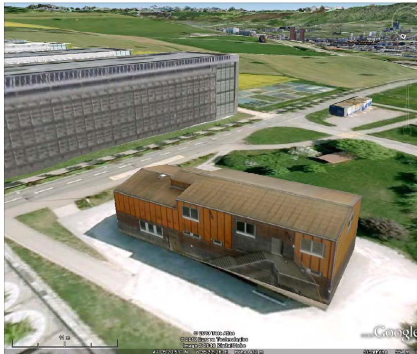
3D-Model derived from UAV images of the HXE-building at Campus Science City ETH Hoenggerberg, imported to Google Earth
