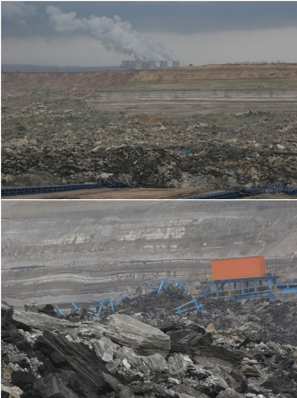
Figure 1: Overview of a real-world accident where a complete daylight coal mining site has collapsed. Several people have been killed and many objects have been buried.
