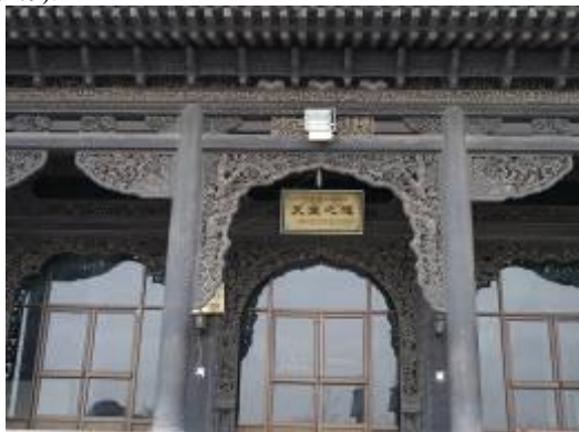
Figure9: decorated brace of Banqiao Mosque
